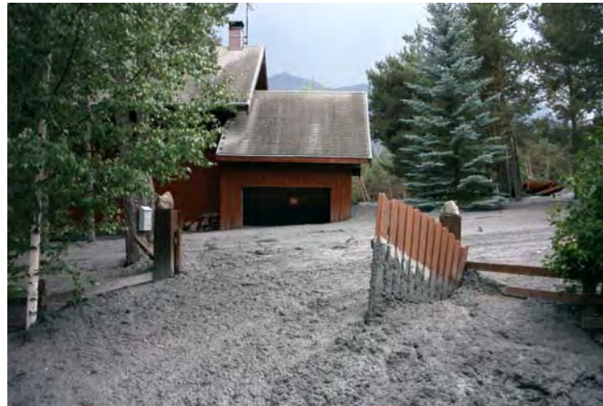
Figure 19: damaged house nearby the torrent
